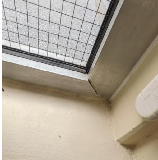
Figure 6 Window in Anzac Room with defective seal in the corner.
