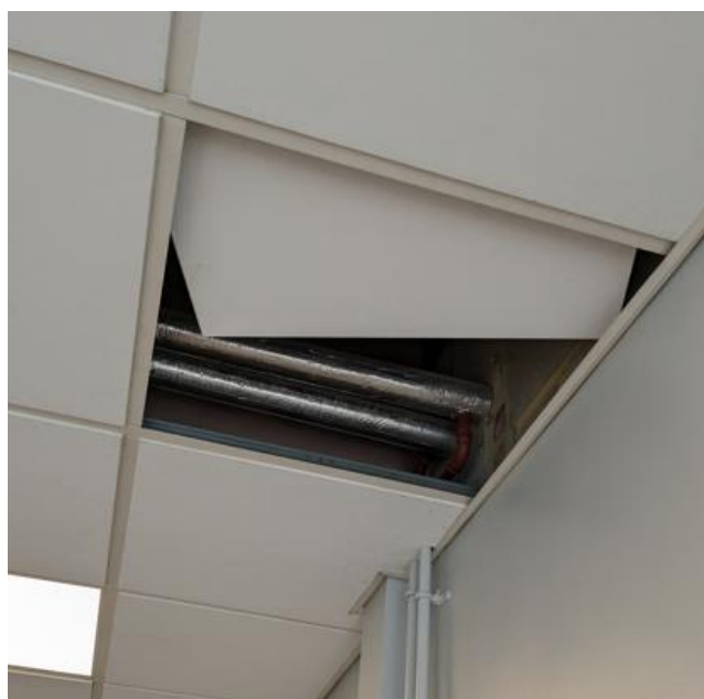
Figure 5 Displaced ceiling tile above entrance corridor – pipes are however lagged.
