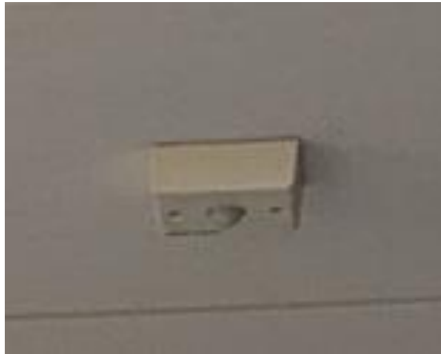
Figure 8 Example proximity sensor in the ladies' toilets.
