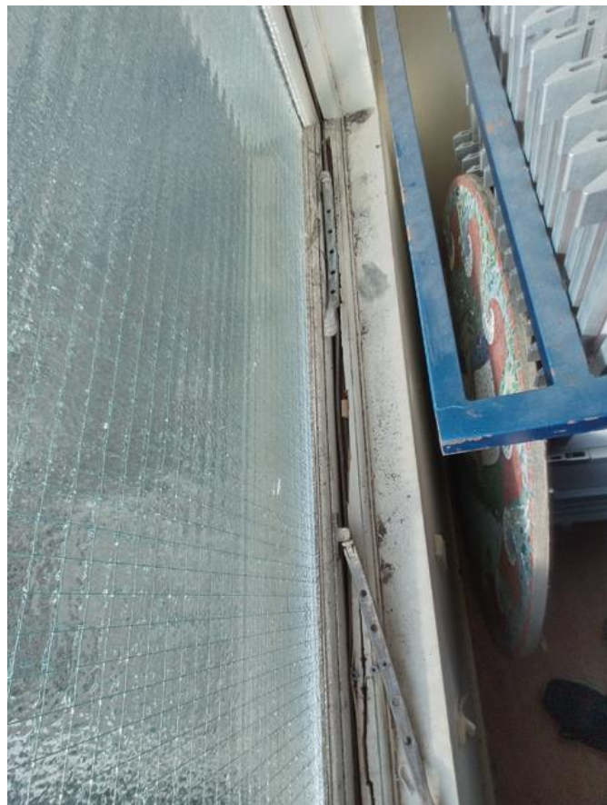
Figure 7 Cracked frame of the Sound Room window.
