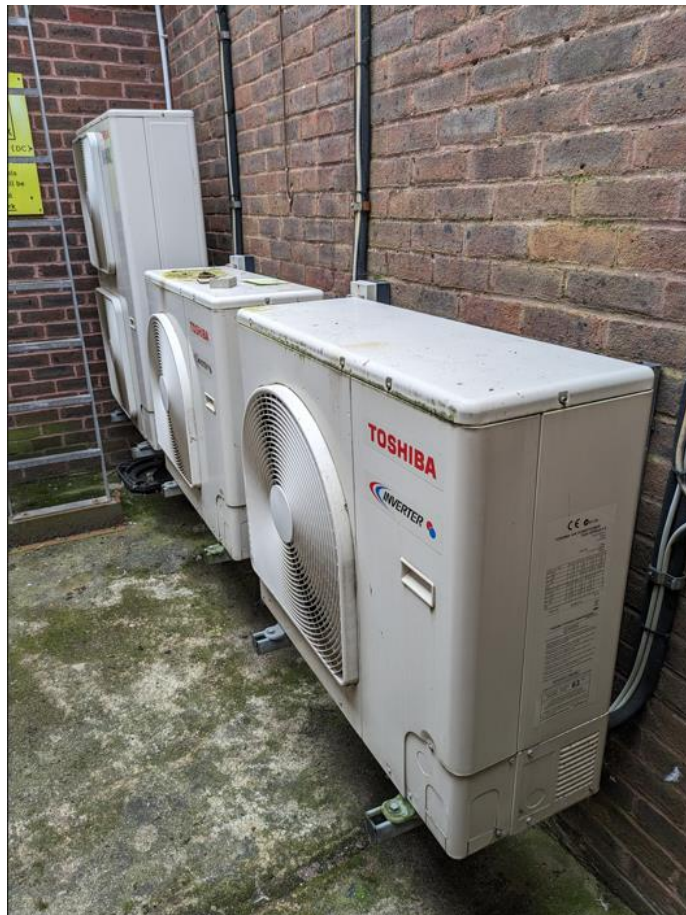
Figure 12 Existing air conditioning units (external components).
