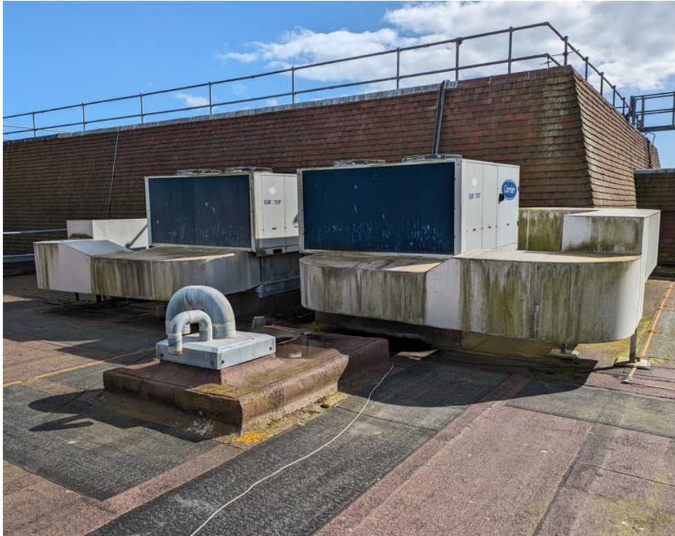
Figure 14 Carrier packaged HVAC units serving the Main Hall.
