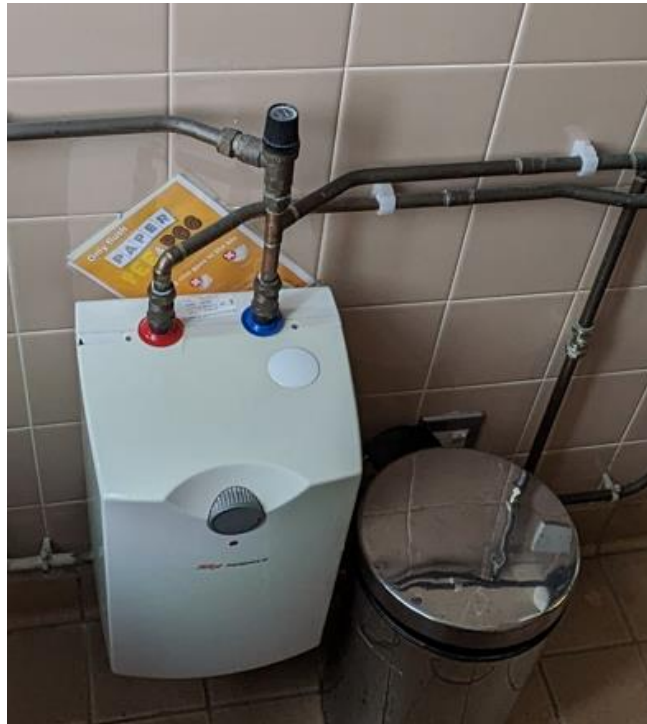
Figure 10 Instantaneous heater in men's toilet by the Robson-Fields room.
