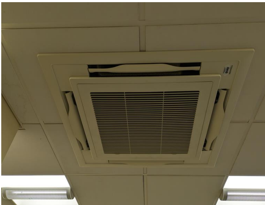
Figure 13 Toshiba ceiling cassettes.
