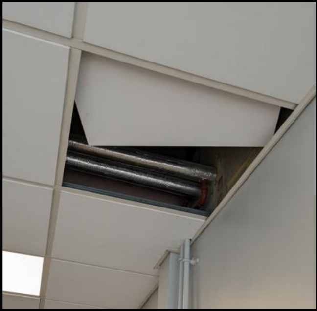
Displaced ceiling tile above entrance corridor
