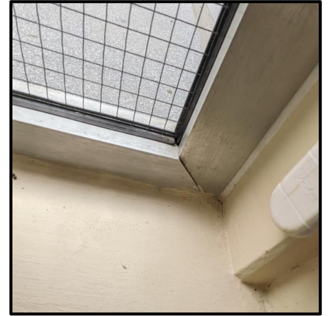
Window in Anzac Room with defective seal in the corner
