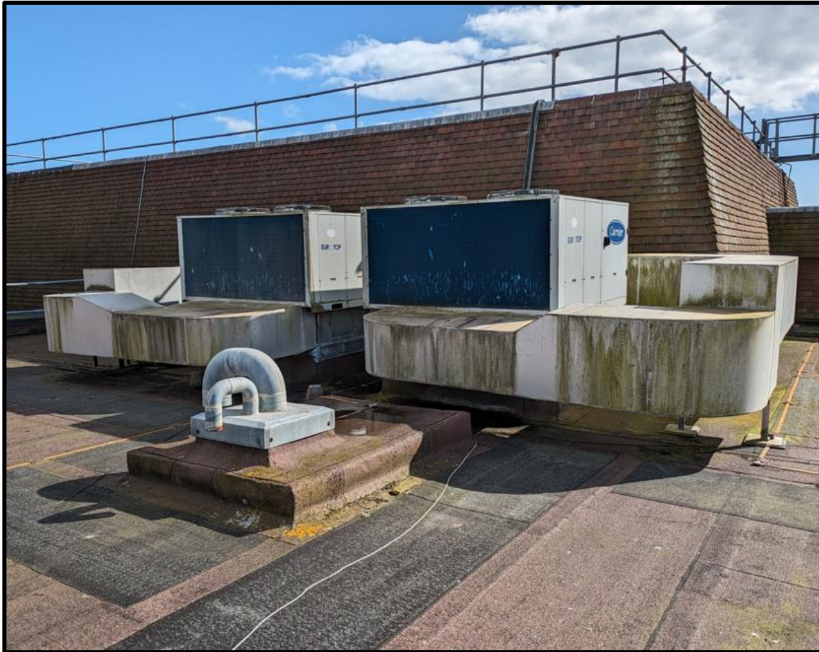
Carrier packaged HVAC units serving the Main Hall
