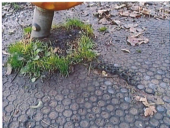
General site – safety matting silted up and does not conform to requirements
