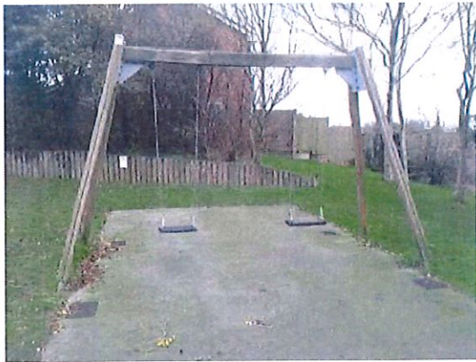
General site – safety matting silted up and does not conform to requirements
