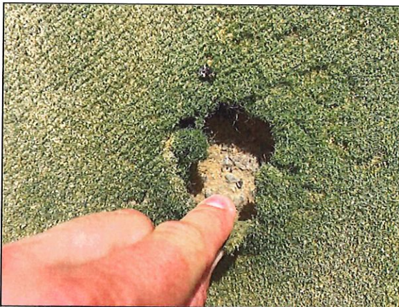
Figure 2 – rips and tears to the surfacing
