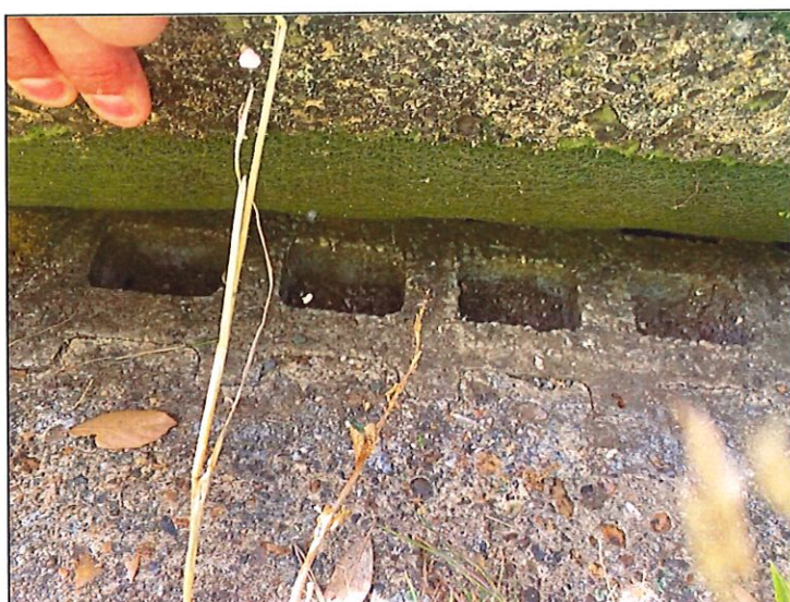
Figure 3 – concrete open block channel to the surrounds
