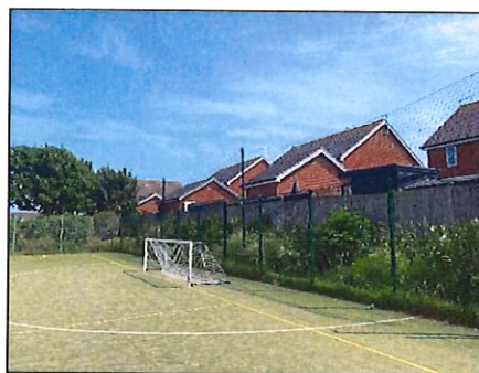
Figure 5 – panel weldmesh fence
