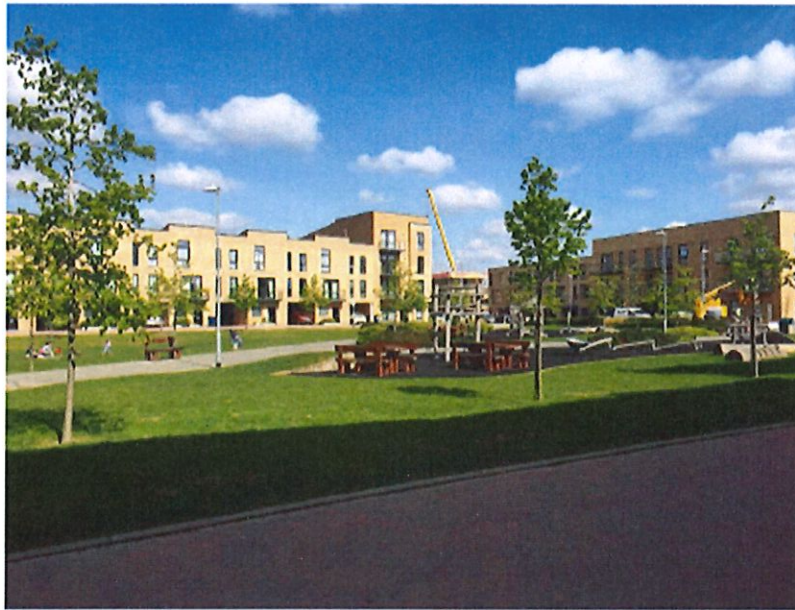
Figure 7. Example of play area incorporated within and around a SuDS basin feature (Img. Basin01).
