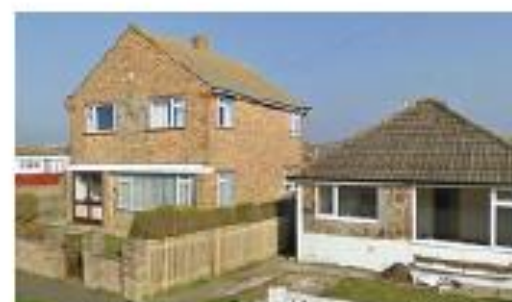
Figure 34. 2 storey dwelling adjacent to a bungalow.
