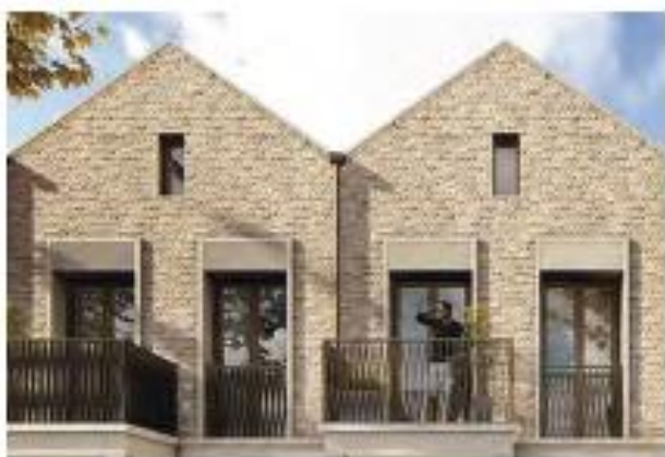
Figure 234. M shaped roof.
