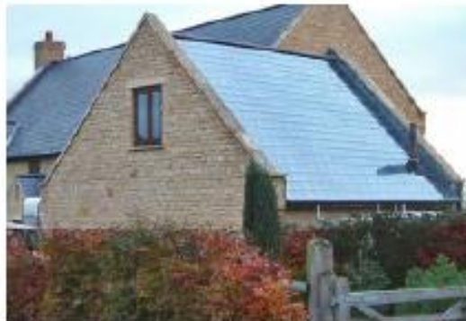
Figure 323. Solar panels integrated sympathetically with a traditional building.
