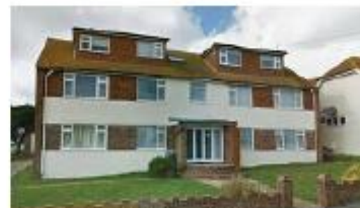
Figure 36. Tallest buildings within the Coastal Plotlands are 2.5 storeys.
