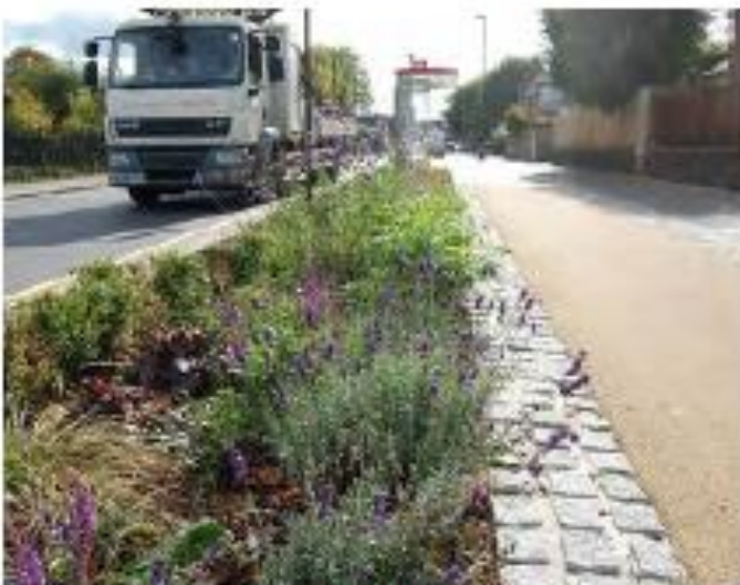
Figure 176. Planted verge as part of a rain garden scheme.
