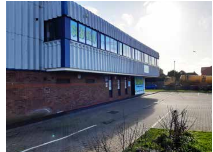
Figure 8: Industrial unit converted to a trampolene park.
