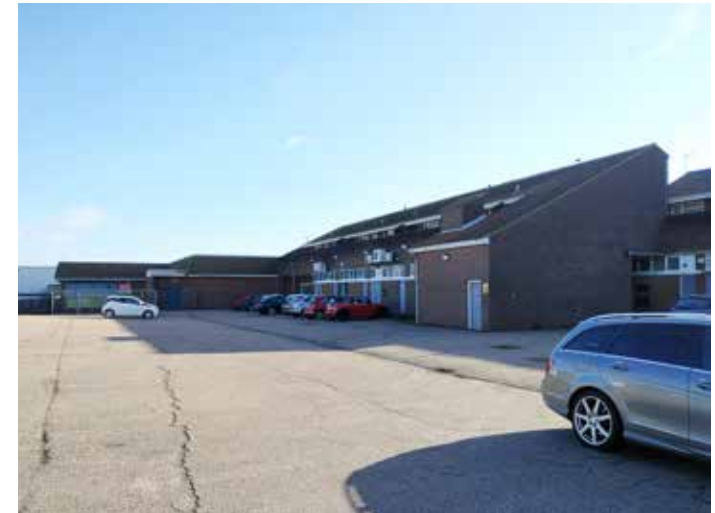
Figure 13: Service area for Meridian Centre shops with flats above.
