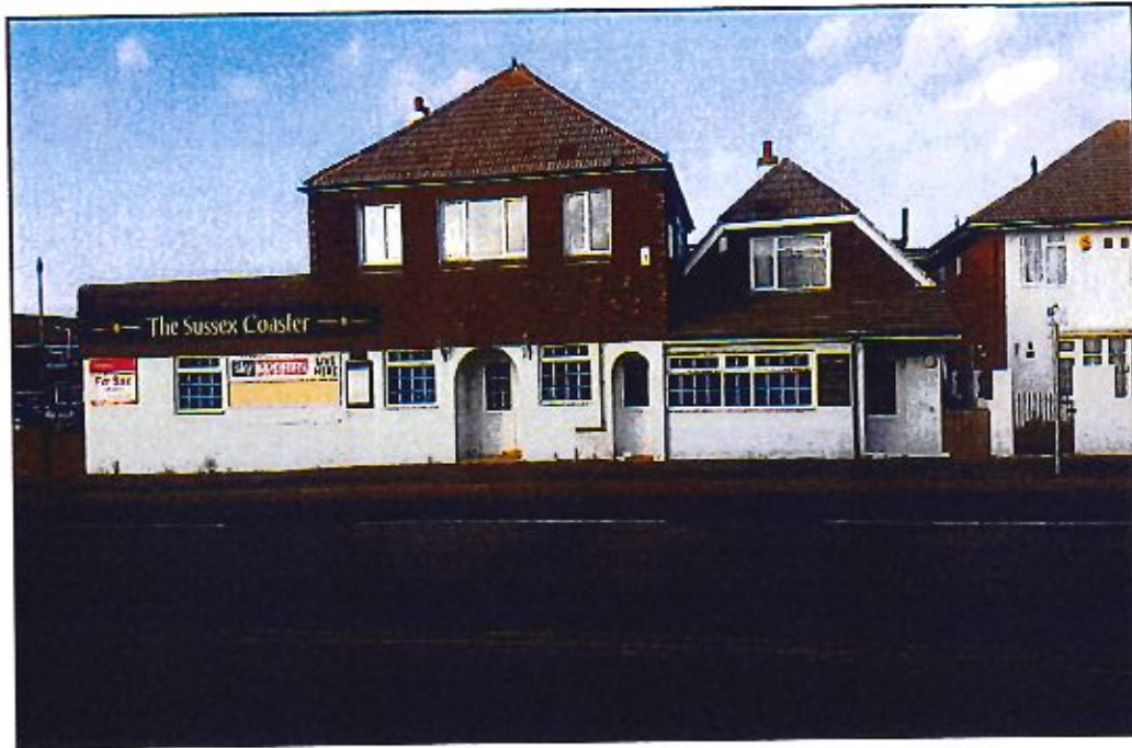
Figure 1: Principal elevation of existing public house
